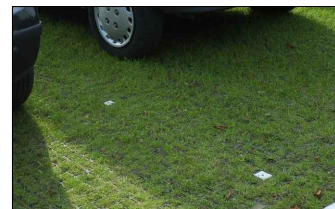
Reinforced Grass Surfacing
