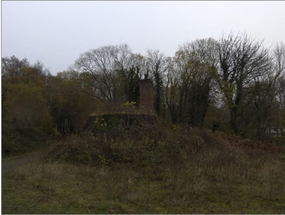
Photograph 26: View east of Brick Kiln and Stack, outside the PDA.
