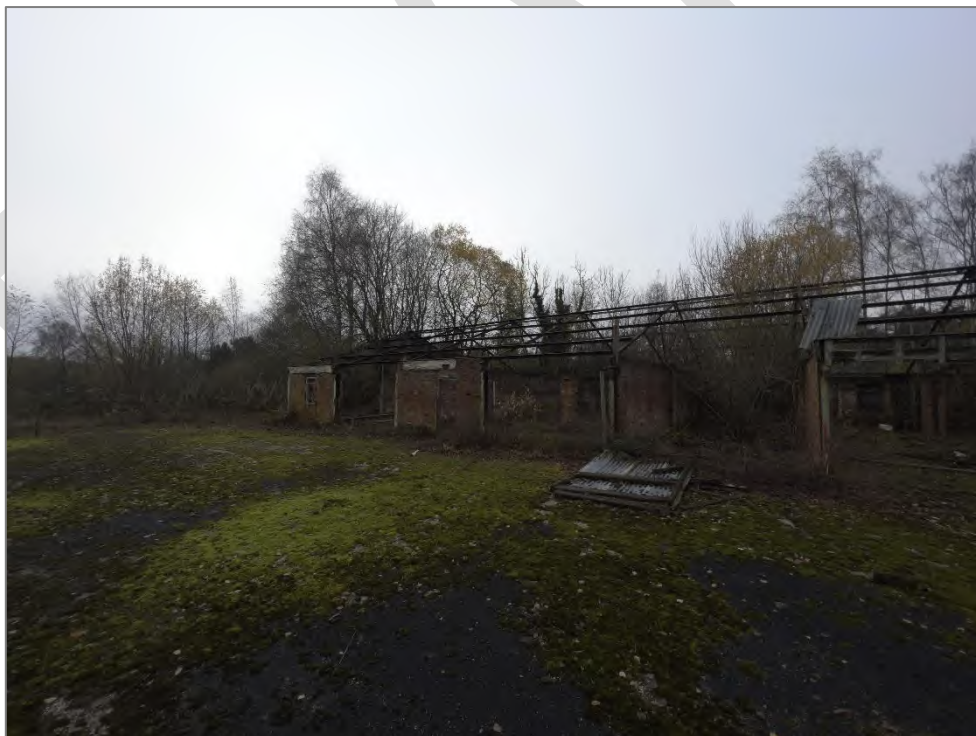
Photograph 8: View southwest towards the late-20th century derelict building.
