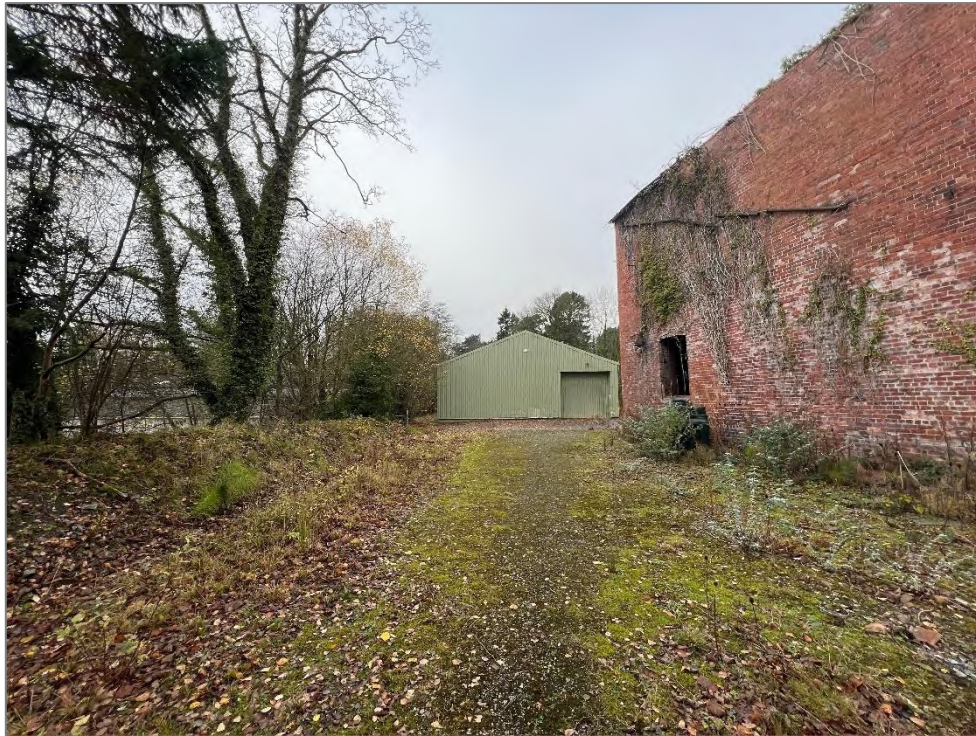
Photograph 3: View west of northern boundary between the PDA and Ore Shed.
