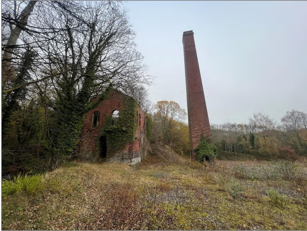
Photograph 17: View northeast towards Taylor's Shaft Engine House and Boiler Stack.
