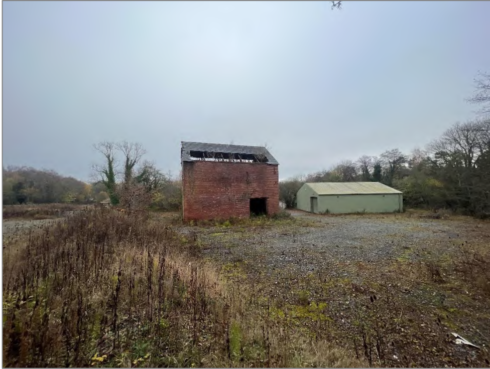
Photograph 20: View west across the soil bund and tree line between the PDA and North Hendre Lead Mine group.
