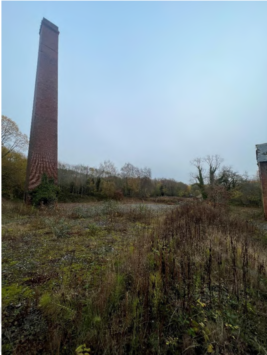
Photograph 19: View south towards the PDA from North Hendre Lead Mine group.
