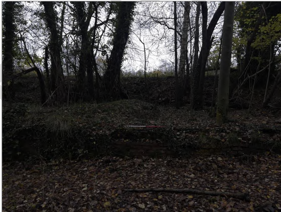
Photograph 16: View View west of possible brick structure/foundations just beyond eastern boundary of the PDA (1x1m scale).
