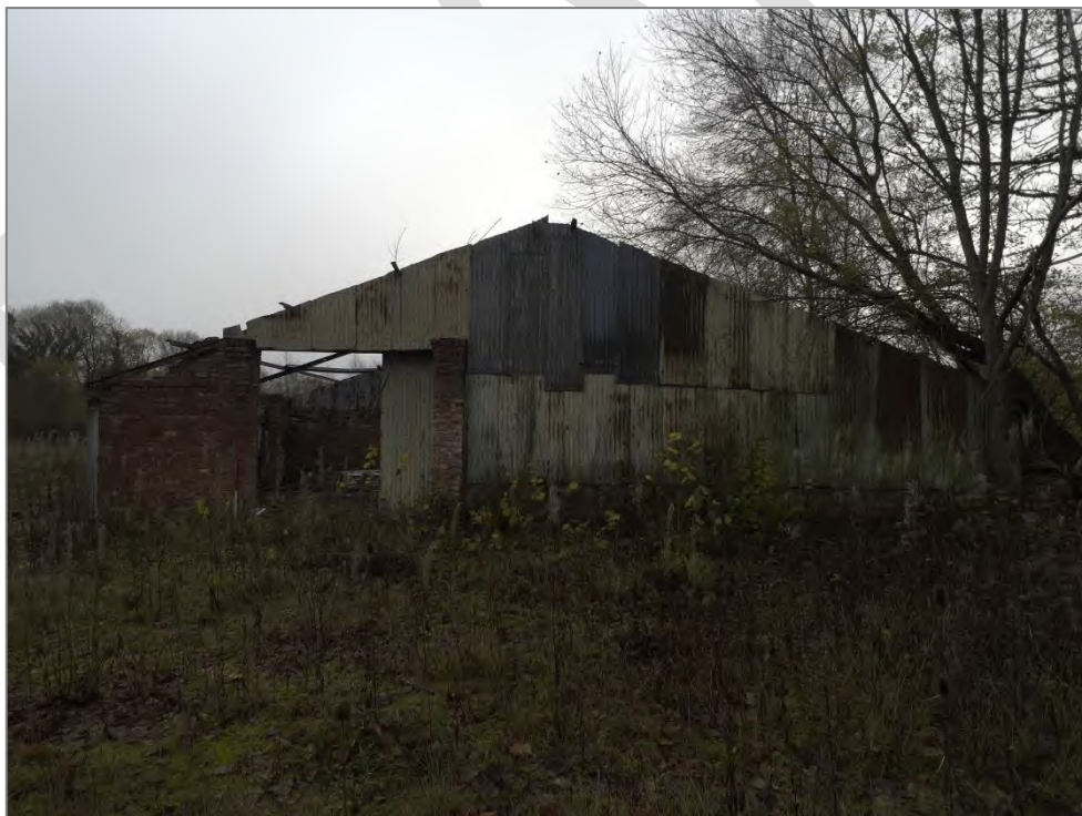
Photograph 6: View south towards the late-20 th century derelict building.
